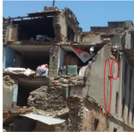
Fig. 3.b: Vertical crack
