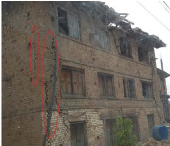
Fig. 3.a: Vertical crack
