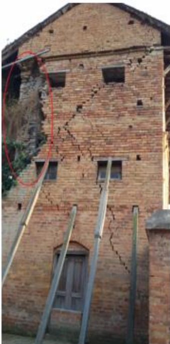
Fig. 2.c: Corner failure
