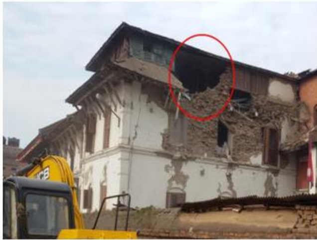
Fig. 4.a: Out of plane failure of top floor
